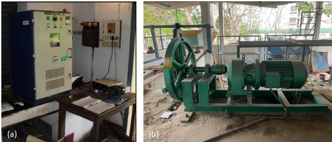
Plate 3.1: Photographic view of (a) Inverter drive and (b) motor
