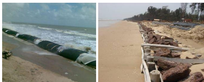
Fig. 2.7 Geotextile tubes at Shankarpur (Sundar et al. 2009).
