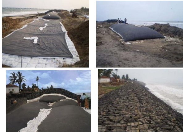
Fig. 2.11 Construction stages of seawall at Uppada, Andhra Pradesh, (Sundar 2013).
