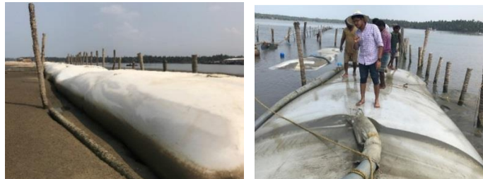
Fig. 2.13 Geotube island reclamation, Cheruvattor, Kerala (photographs taken during field visit)
