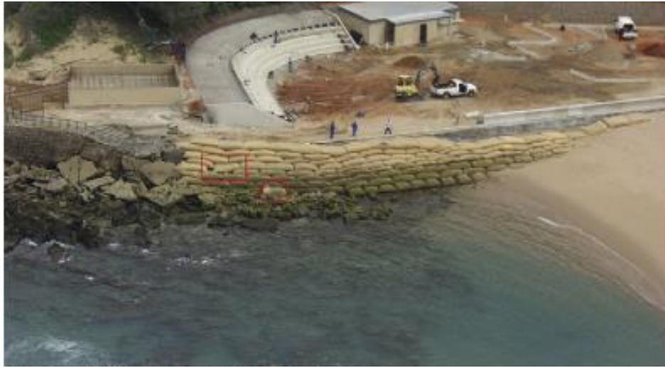
Fig. 2.1 Geotextile bag seawall at Ispingo, South Africa (Corbella and Stretch 2012)
