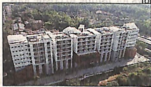
ADDING FACILITIES: New hostels of NITK, Surathkal
