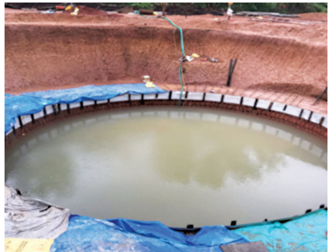
Progress as of 30 June 2020
