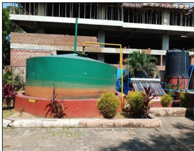
Figure 3.1: Biogas plant near Urwa ground, Mangalore
