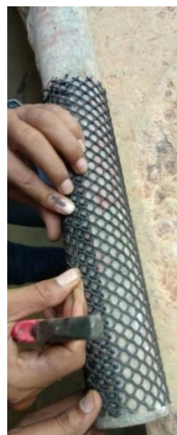
Fig. 4.6 Encasing the casing pipe with geogrid material
