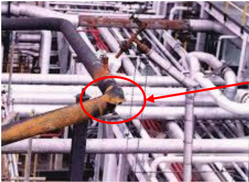
Figure 1.3 Catastrophic failure of an overhead pipeline
