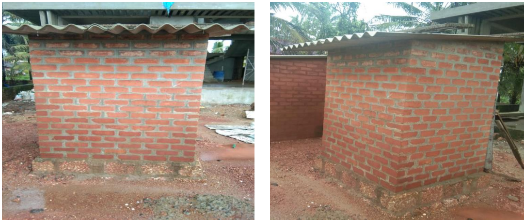
Figure 3.9 A view of model room constructed with ordinary bricks
