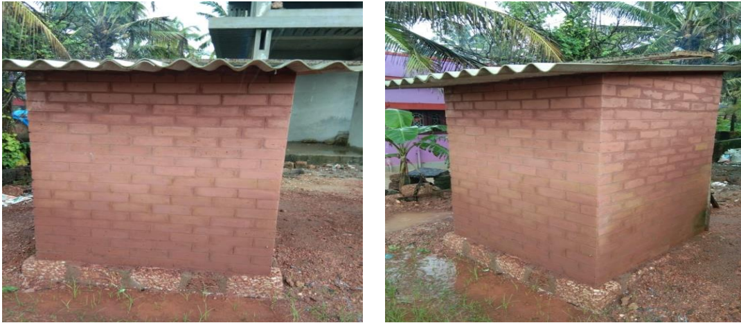
Figure 3.8 A view of model room constructed with IOT and perlite mixed bricks
