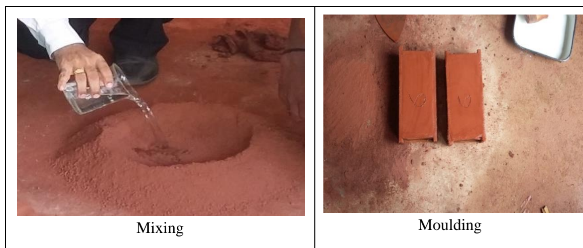
Figure 3.4 A view of casting of bricks
