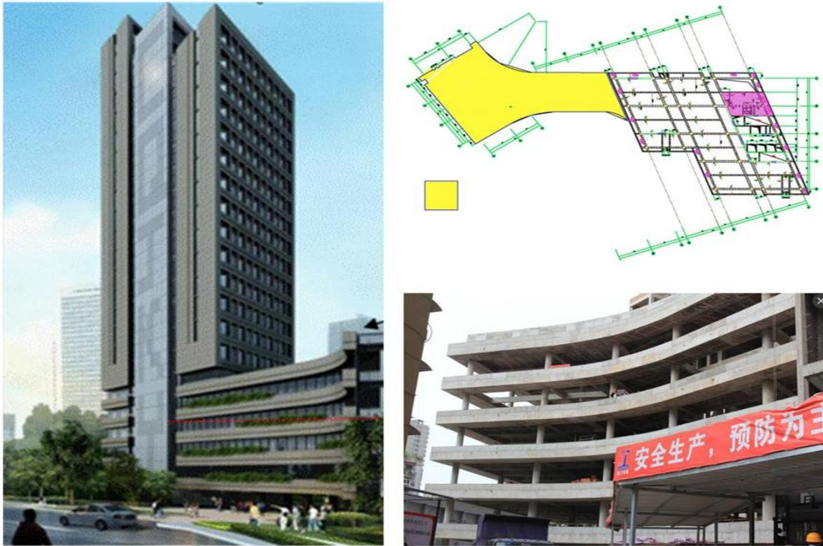
**Fig 2.3 First full scale structural application of alkali activated slag concrete**
