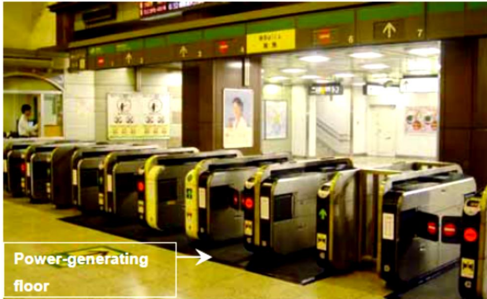
Fig. 2.12 Power generating mats in a JR east railway station (Anon, 2008b)
