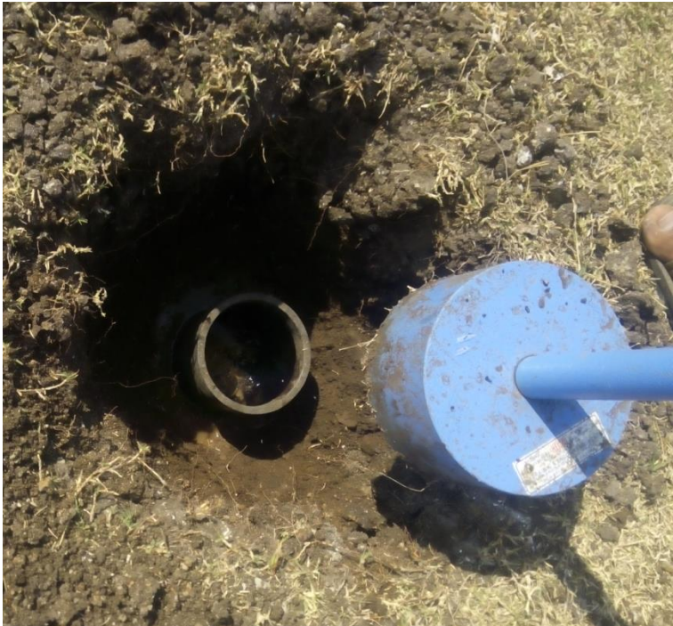
Fig 3.4 Cylindrical sampler (container) being driven into soil to collect the soil sample after the in situ test
