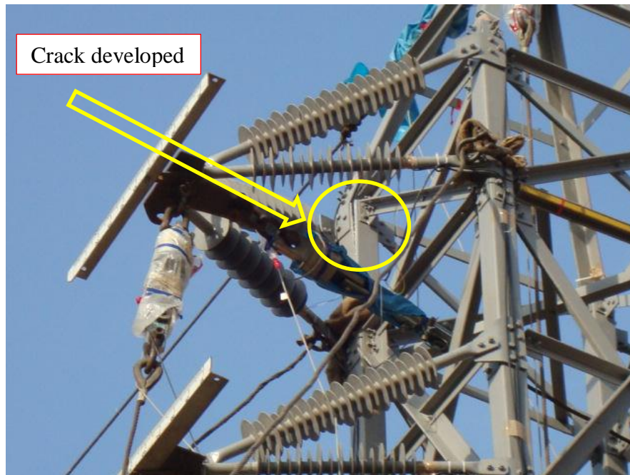
Fig. 4.22a Cracking of leg member at the base of top cross arm
