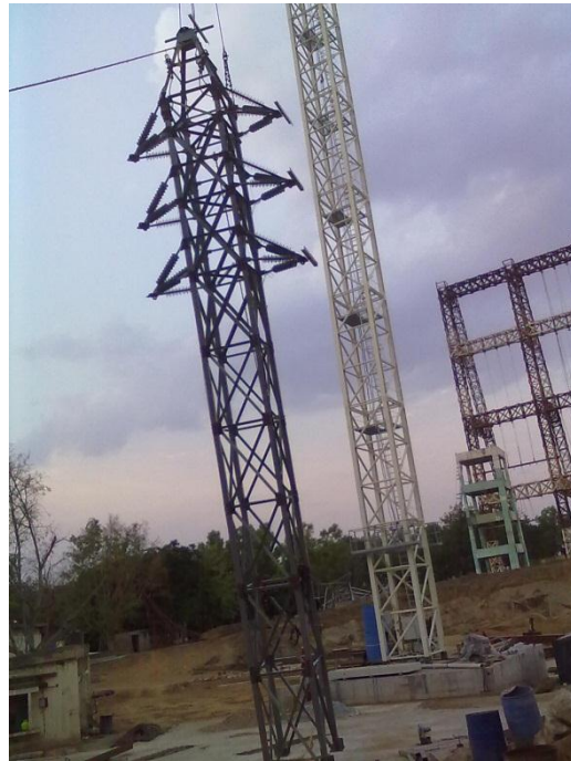
Fig 3.30 Photograph showing constructed full size (15 m) tower with composite members.
