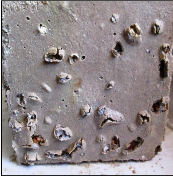
(a) Cube sample after aggregates undergo expansion leading to pop-out of surface
