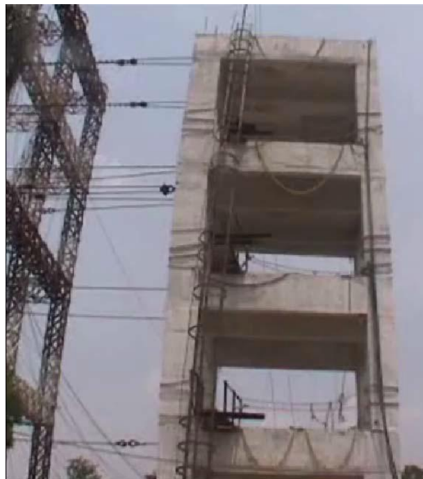
Figure 3.10 Structure during the test
