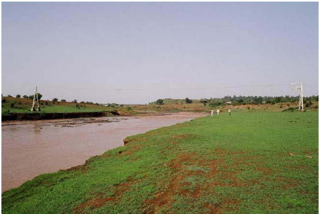
Figure 3.2. Gilgel Abay Hydrometric Station (Field visit photo)
