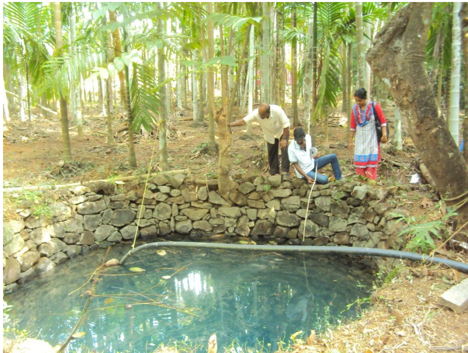
Fig.3.5 Photograph of pumping well no PW1
