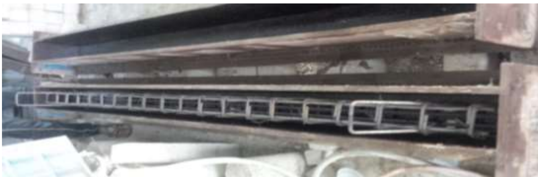
Fig 3.4 Formwork for beam specimens
