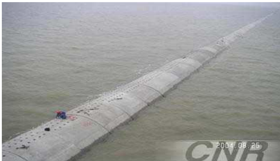
Fig. 2.4 Semicircular breakwater in Yangtze River Estuary, China
