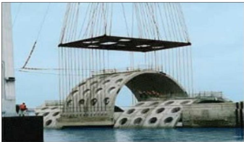
Fig. 2.2 Lowering of semicircular breakwater caisson from a floating crane
