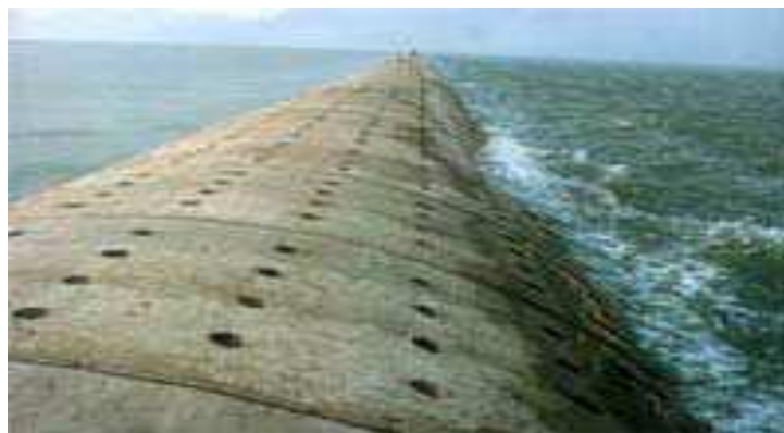
Fig. 2.3 Semicircular breakwater in Tianjin Port, China
