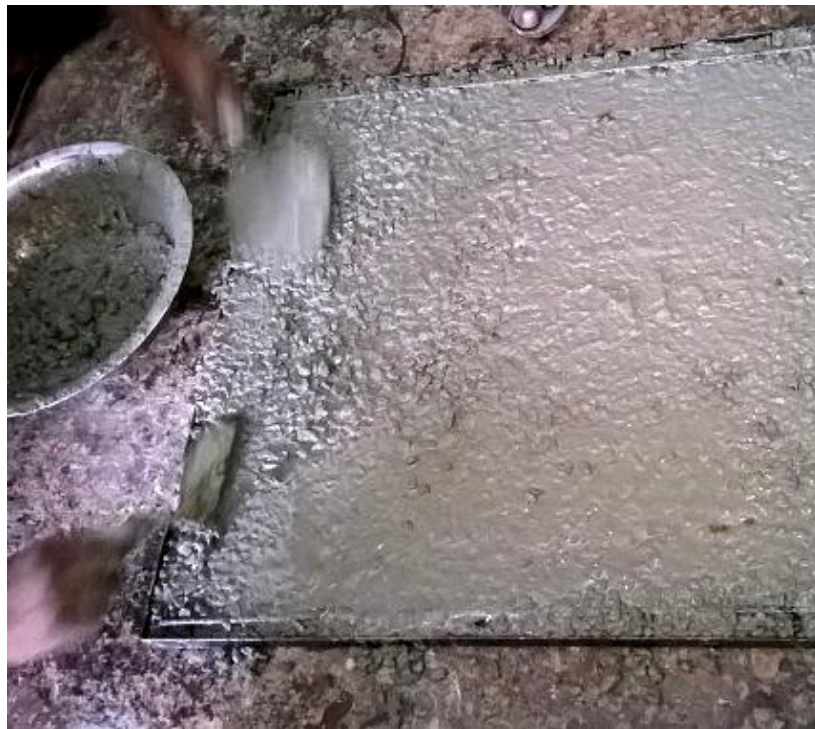
Plate 3.3 Preparation of the base slab
