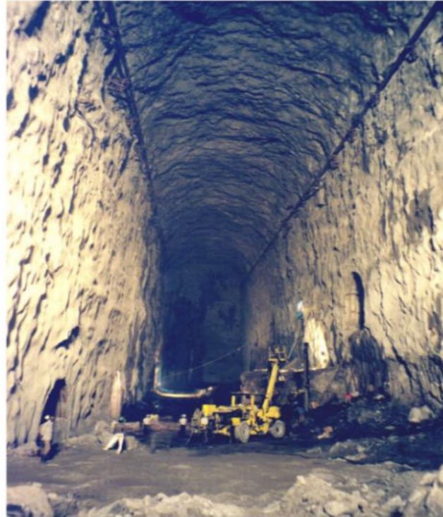
Fig. 2.3 Powerhouse cavern of Nathpa Jhakri hydro electric project, Himachal Pradesh (Hoek, 2000)
