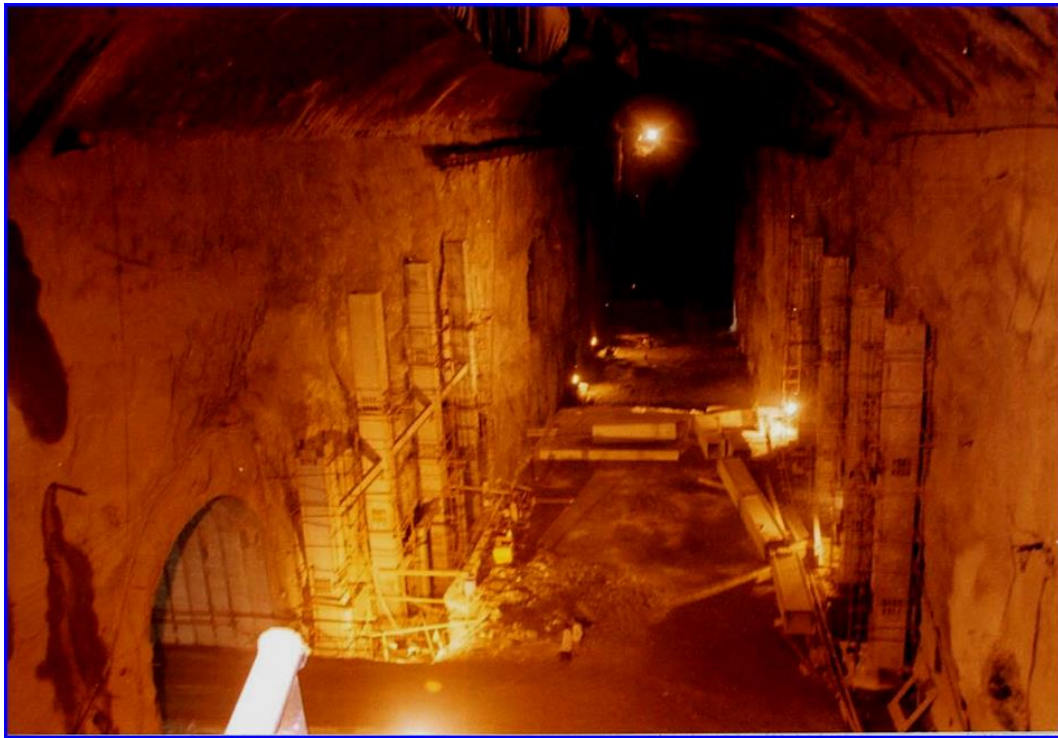
Fig. 3.9 Powerhouse cavern after complete excavation, Tala Hydroelectric Project
