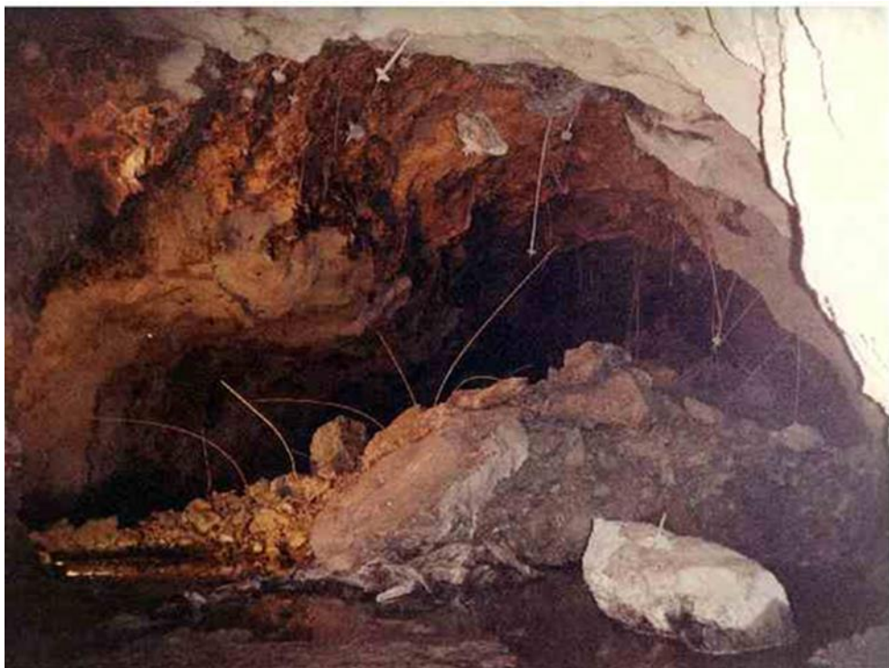
Fig. 4.9 Roof collapse at powerhouse cavern
