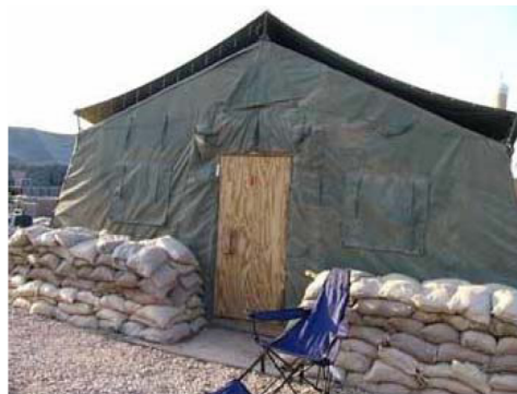
Figure 14 Usage of sand bags for guarding security posts (see online version for colours)
