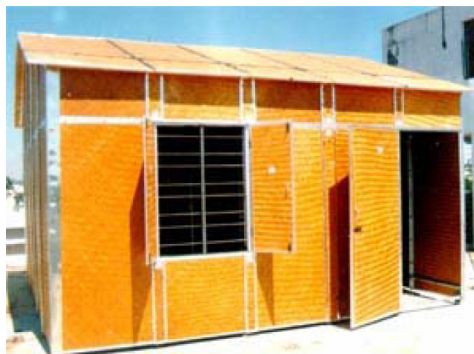
Figure 15 Sandwich structure as a replacement for sand bags (see online version for colours)
